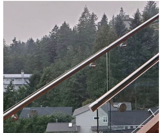
Finished Installed Railing
